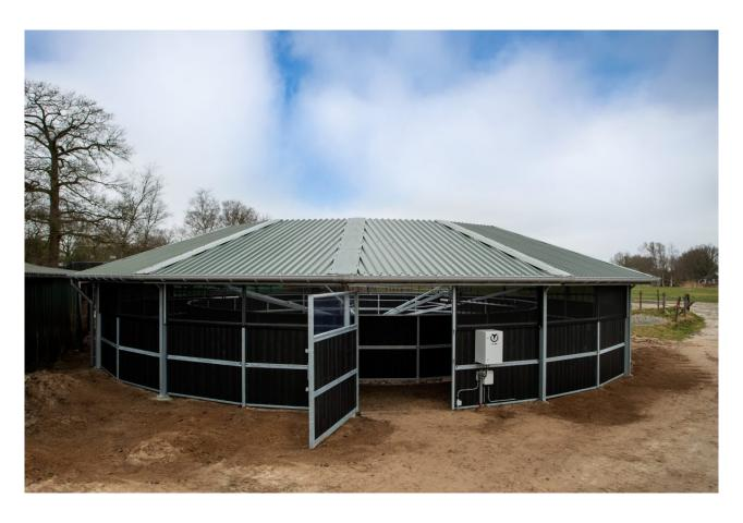
Our sustainable steel fencing for track roofs and Ifull roof covers, crafted with high-quality steel C-profiles. Each truss section is equipped with 2 fencing sections, which can be filled according to your preference with plastic boards, pressure-treated wood boards, or hardwood planks. Explore the versatility and quality of our fencing options for a stylish and functional addition to the roof.
