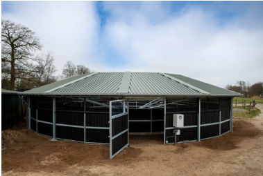
Fencing for a 16-meter roof
