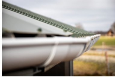
Rain gutter 14 sections
