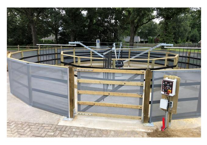
Windbreak mesh around the outside of the fence. The windbreak mesh is tensioned by a tension roller at both ends. The windbreak mesh is hemmed over the full length and is secured all around with a clip to prevent sagging.
