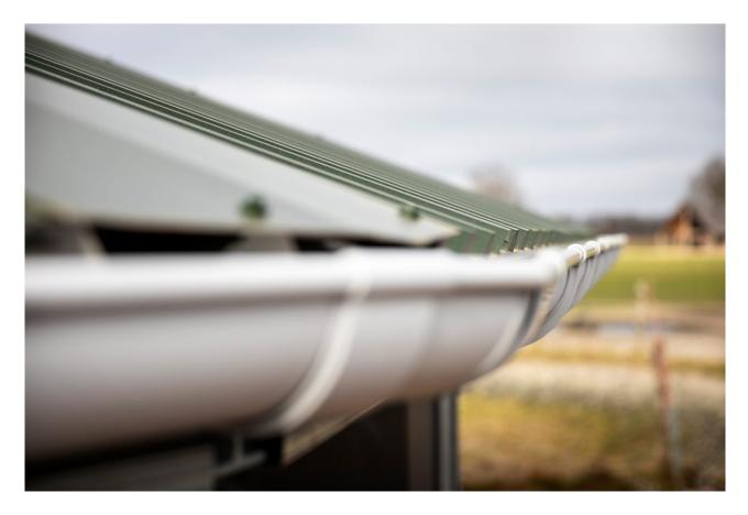
Plastic gutters around the roof. Consisting of mast gutter 170mm. Max 3 sections connected together. The drain runs to ground level.
